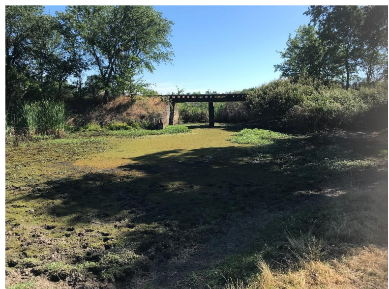
4. North Fork Badger Creek at Railroad trestle
