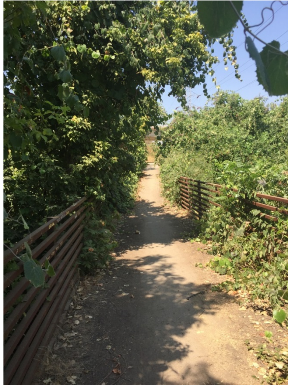
Exhibit 6 – ND3B – Bridge – 10’ wide (Department of Regional Parks, June 2017)
