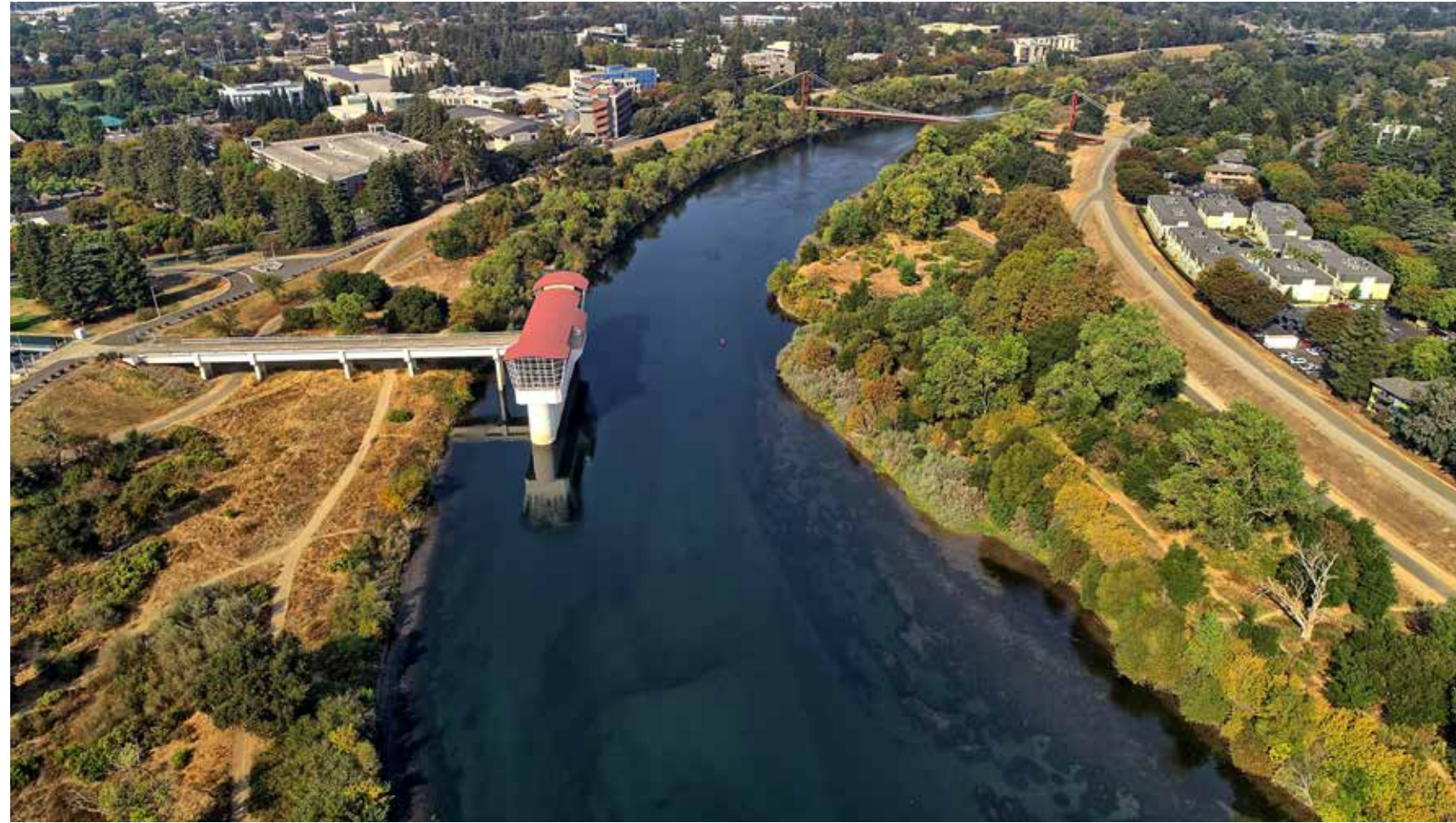
Aerial view of the E.A. Fairbairn Water Intake Station and Guy West Bridge in the Campus Commons Area. Photo Credit: Regional Parks
