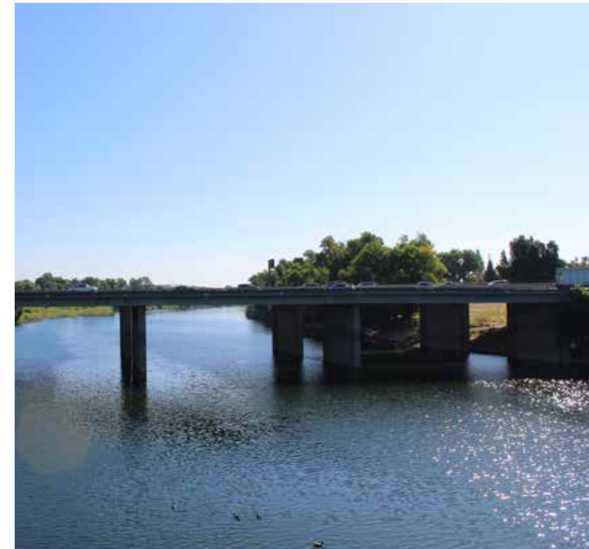
The I-5 American River Bridge in the Discovery Park Area. Photo Credit: MIG
